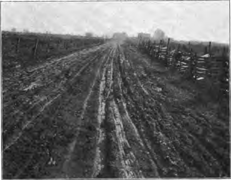
Elmer and Alloway road, Salem Co., before improvement.
